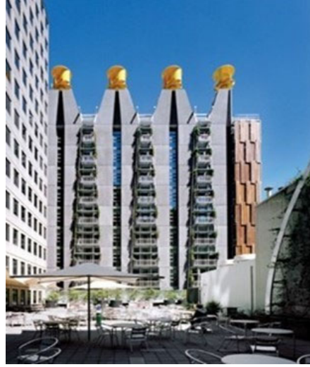
Şekil 6. CH2 Melbourne City Council House 2 [26]
